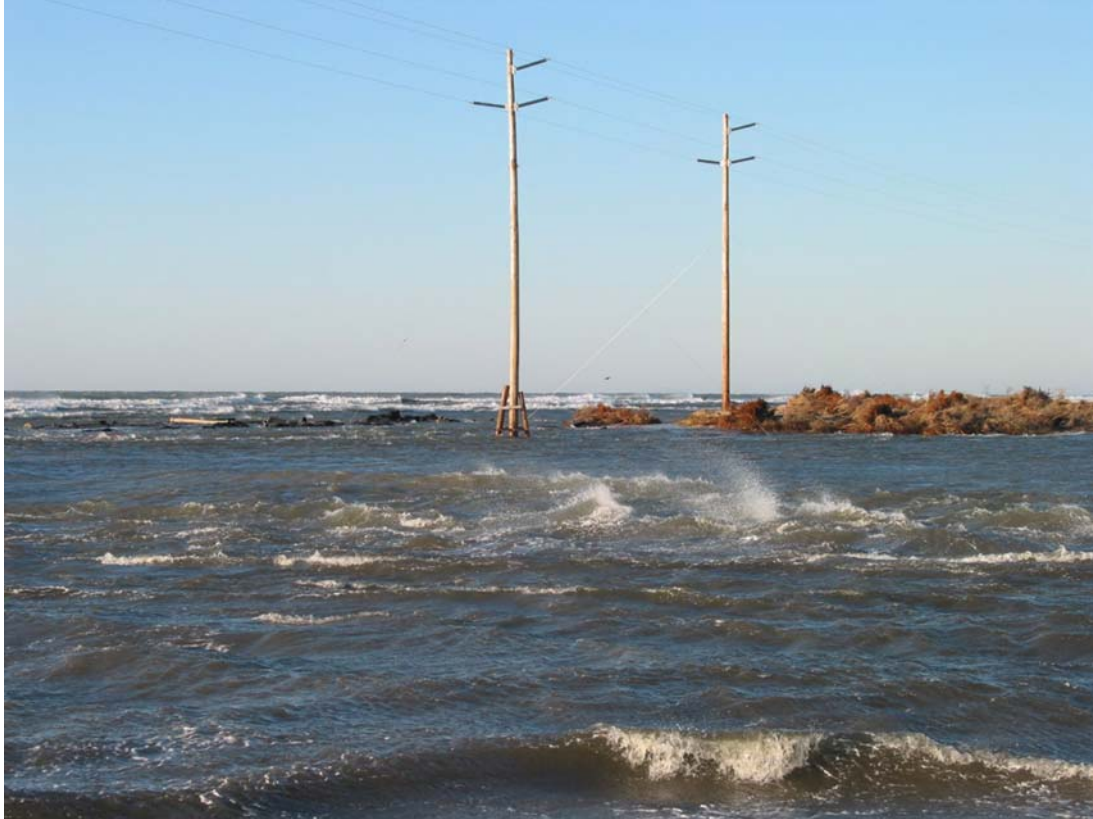
Figure 5. Photograph illustrating high velocity tidal currents, wind-driven currents, and waves within the main breach channel.
